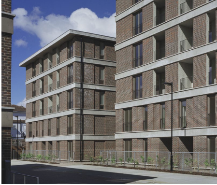
Finsbury Park, Finsbury, London Sergison Bates Architects
