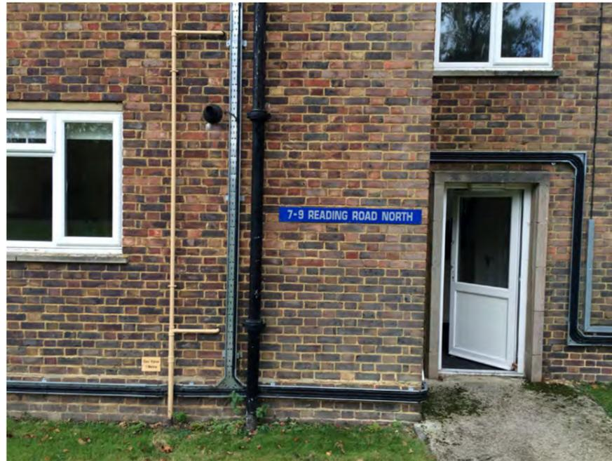
Service pipes and cables visible on the exterior of the buildings are unsightly and indicate poor design.
