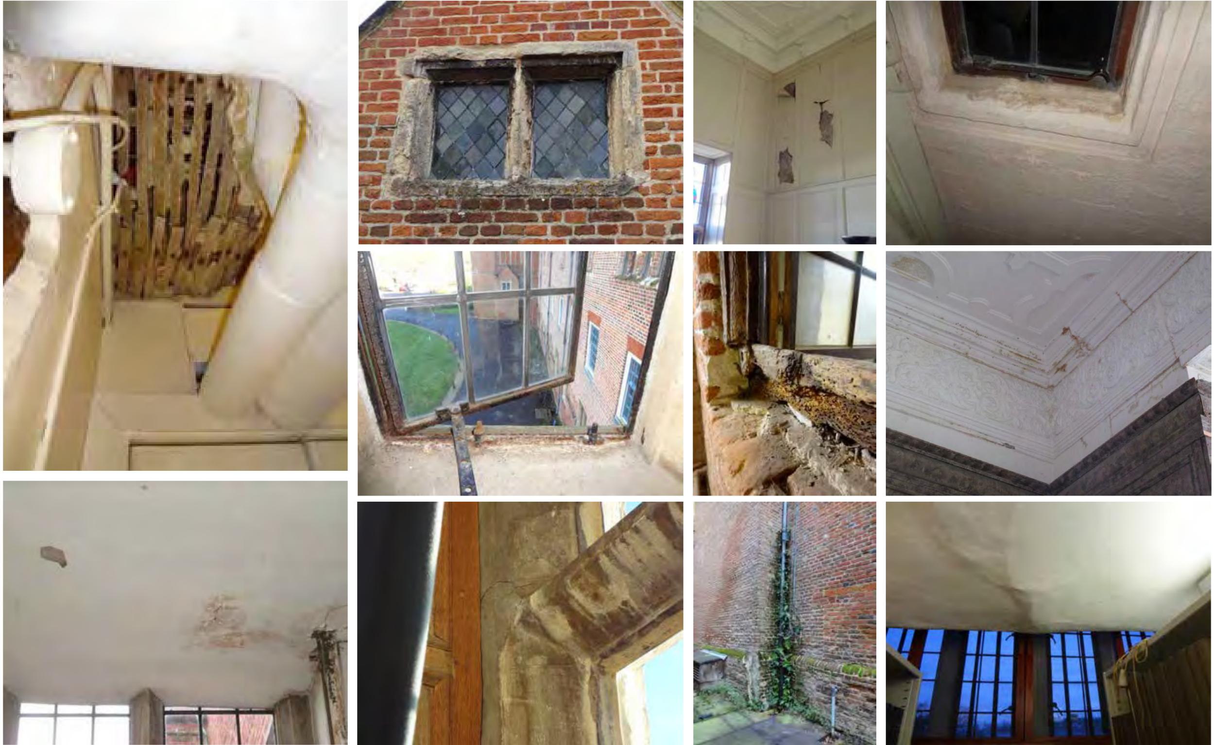
PHOTOGRAPHS SHOWING INTERNAL DAMAGE FROM WATER PENETRATION, STRUCTURAL MOVEMENT AND WEATHERING
