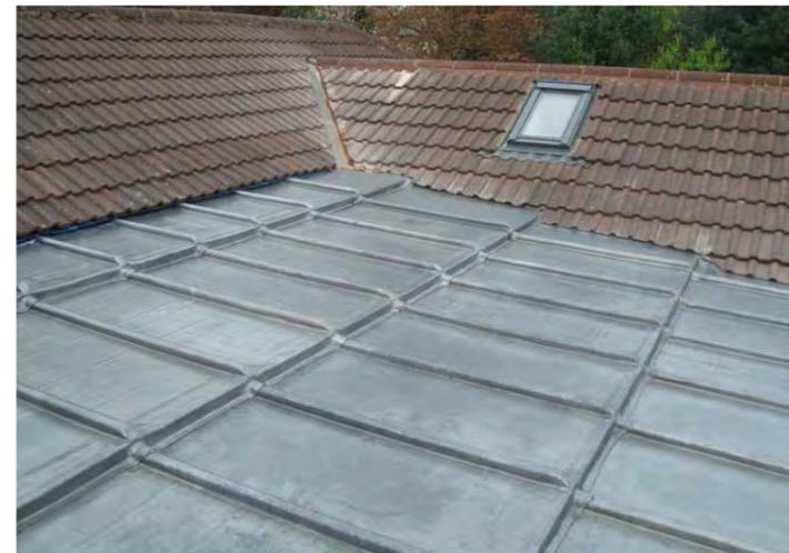
Example image showing lead roofing
