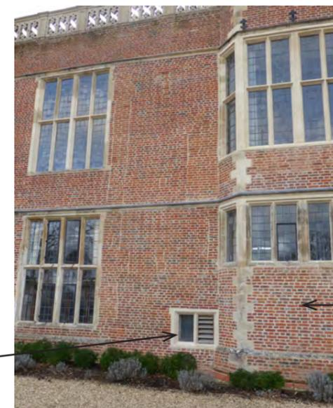
Existing vent to be replaced with window
