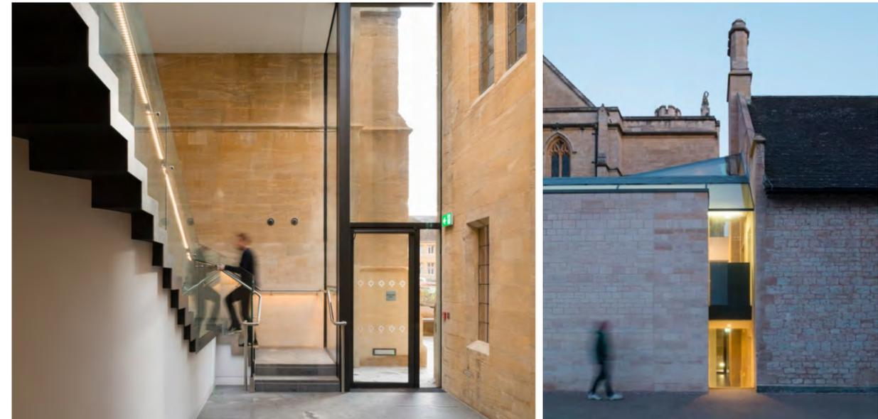
Example images showing how the junction between new and old can be managed sensitively and innovatively, particularly when integrating new access and circulation to historic buildings such as stairs, glazed screens and lifts. <http://www.batstudio.co.uk/East-Range-Mansfield-College>
